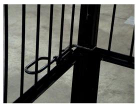
Install the door latch as shown with the provided hardware.
