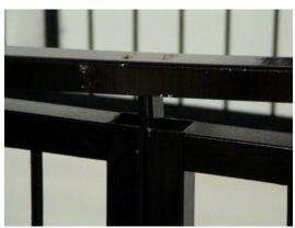
Insert the wall stiffener so each leg of the stiffener bracket slides into the modular panel frame.
