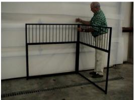
Install a panel connect in the top of the two panels to secure them in position. Continue to install back and side panels in the same manner in the position required.
